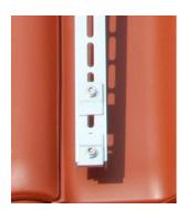
Tighten the toe bar between the clamps und fix it by tightening the screws.
