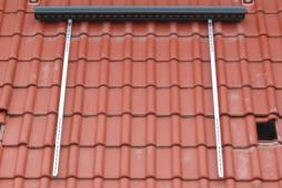
Take the lower part of the toe bar (3) and arrange it centrally on the side bars (2).
