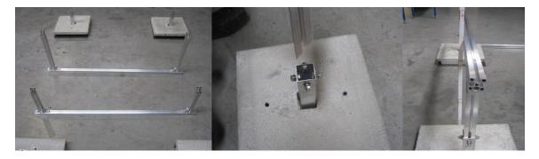
Connect the longitudinal rails of the toe and manifold side with the profile rail set ST-ADM-3.3P (1900 mm) and the profile angle set ST-ADM-2BW to a rectangle. Insert the screws M8x40 into the longitudinal rails and fit the spacer (Fastening set ST-ADM-2BM).
