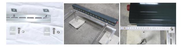
For the installation of the toe bar, mount the clamp in the 1st and 3d punching at the lower part of both bars by using one hex socket head screw M8 x 25, one lock washer M8, one clamp and one cage nut each. Screw the clamp loose. Put the toe bar on top and install the tubes on the left and on the right. Then arrange the manifold case and toe bar parallel to each other. Tighten the clamps.
