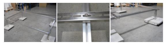
For the installation of the manifold case, mount the clamp in the 1st and 5<sup>th</sup> punching at the upper part of both bars by using one hex socket head screw M8 x 25, one lock washer M8, one clamp and one cage nut each. Screw the clamp loose. Put the manifold case on top and arrange it centrally. The side bars should be positionned between the second and third tube. Then tighten the clamps.
