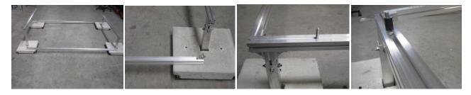
Mount the module side bars (U-profile) and fix them loose with washer and nuts (Fastening set ST-ADM-2BM).
