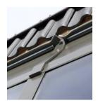
Fix side sections and upper covering sections of mounting frame to the battening with sheet fixing hooks, screw on side sections and upper covering sections of mounting frame (sheet metal screw  $3.5 \times 16 \text{ mm}$ ).
