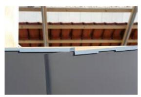
Slide the **batten brackets** and **snow load brackets** into the cut-outs and screw them on (chipboard screws 5 x 35 mm). For an optimum alignment of the batten brackets we recommend fixing a taut string line between the first and the last batten bracket as a guideline.
