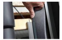
Replace missing tiles and professionally cut to size if necessary. Remove film from self-adhesive roof connection strip and mould strip to shape of tiles.
