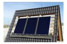
Fit, lock into place and align bottom sections of mounting frame.
