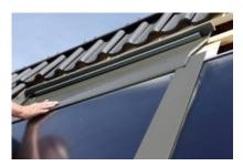
Put sealing tape on the **mounting frame connection strips, short**, hook them in and screw them on (screw with attached washer 4.5 x 35 mm).
