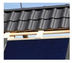
Fit, lock into place and align upper covering sections of mounting frame on the left, in the middle and on the right.
