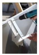
Starting from the left, insert the **flat plate collectors** into the batten brackets and align them so that the gap between the batten bracket and the outer edge of the collector is the same on both sides.
