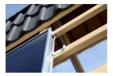
Plug the compression fittings into the collector pipes, mount the other flat plate collectors as described above.
