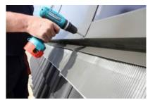
**Bottom sections** and **side sections of mounting frame** are to be connected to each other on the left and right by flipping over the metal plate.
