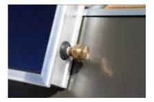
Before the mounting frame is mounted, the collector array is to be pressure tested at 6 bars independently of the rest of the solar installation and the screw connections checked for tightness!
