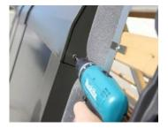
Screw together bottom sections, side sections and connection strips of mounting frame (sheet metal screw  $3.5 \times 16 \,$  mm).
