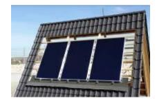
Once all the **flat plate collectors** have been mounted, all the compression fittings (brackets, T-fitting with thermowell, end caps) are to be fitted and aligned. After that, uniformly tighten all the **compression fittings**.
