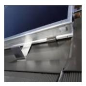
Screw the **flat plate collectors** to the battening on both sides at the top and bottom with **aluminium Z-profiles** (chipboard screw 6 x 60 mm).
